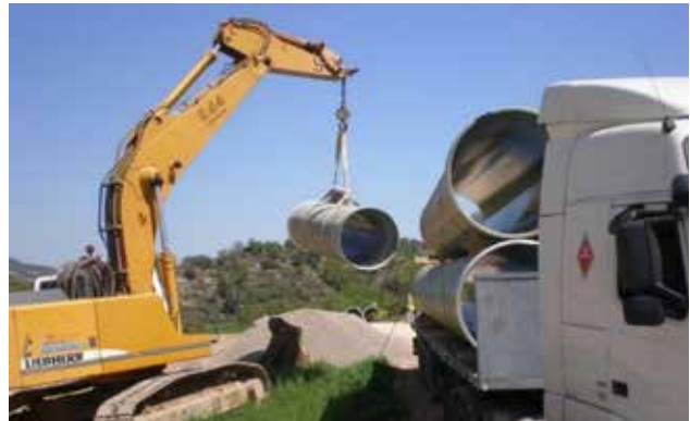
Figure 5 - Lifting Single Pipe
