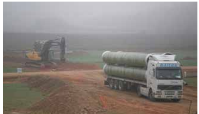
Figure 3 - Transporting Pipes to Site
