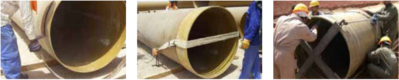
Figure 22 - Mounting the coupler on the pipe
