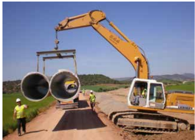
Figure 6 - Lifting Unitized Package
