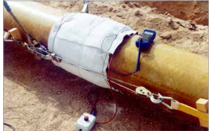
Fig. 5.5. Curing of adhesive bonded joint under tension
