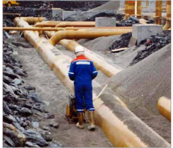
Fig. 6.9. Compaction of backfill material
