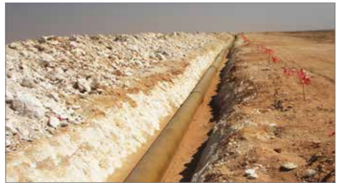
Fig. 6.2. Trench in stable soil
