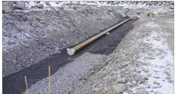
Fig. 6.8. Pipe assembly in process in prepared trench
