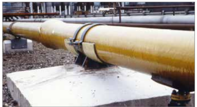
Fig. 7.5. Fixed point with adhesive bonded saddles
