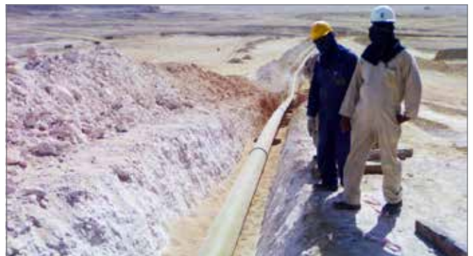
Fig. 6.13. Pipe alignment
