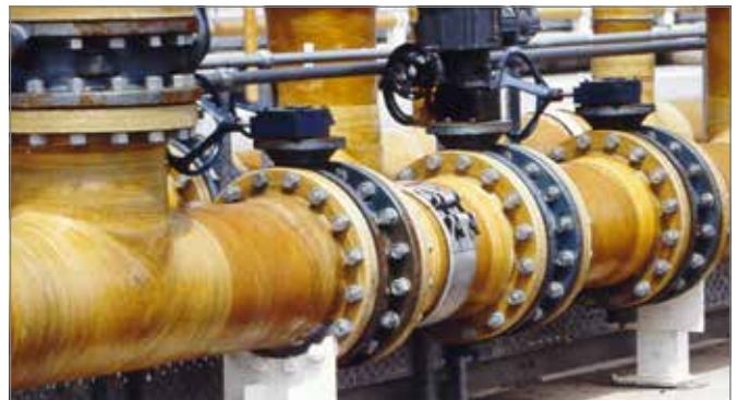
Fig. 4.4. Flange joints
