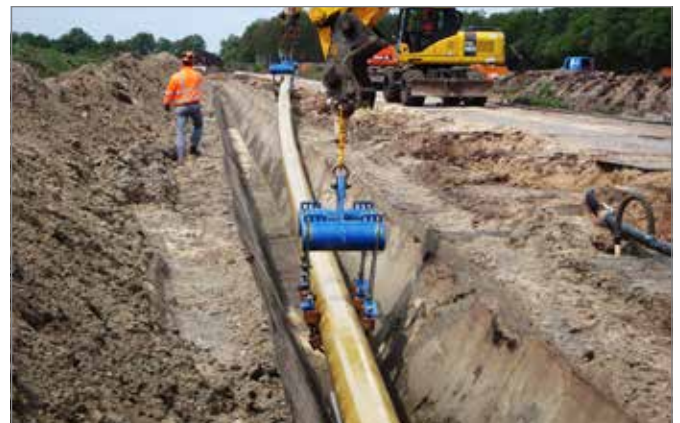
Fig. 6.5. Assembly in the trench
