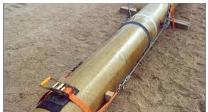
Fig. 5.4. Pulled adhesive joint
