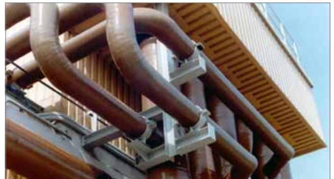
Fig. 7.2. Pipe supports
