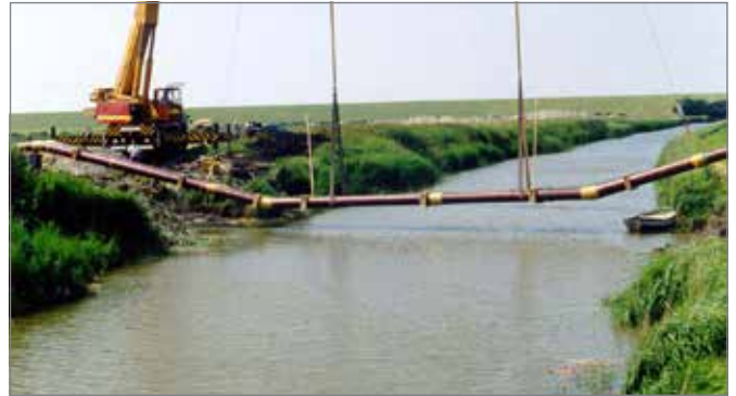
Fig. 6.12. Launching of a channel crossing
