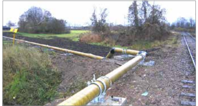
Fig. 7.4. Support with fixed point
