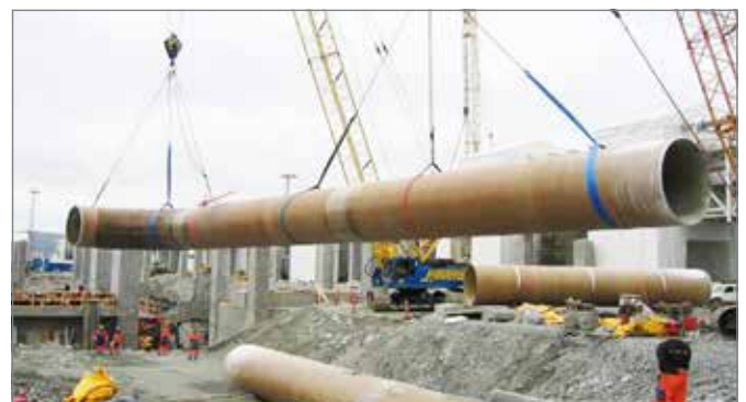
Fig. 3.4. Multiple support spool lifting
