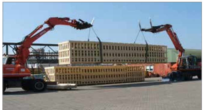
Fig. 3.6. Dual crane handling
