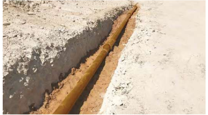
Flowstrong GRE Pipes & Fittings Diameter Range (DN): 3" - 16" Pressure Class (PN): Up to 3000 psi Standard Lengths: 6 - 12 m
