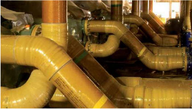
Wavistrong GRE Pipes & Fittings Diameter Range (DN): 25 - 1600 mm Pressure Class (PN): Up to 120 bar Standard Lengths: 3 - 12 m
