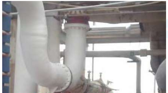
Fiberbond GRP Pipes & Fittings Diameter Range (DN): 2" - 30" Pressure class (PN): Up to 13.8 bar Standard Length: Up to 9 m
