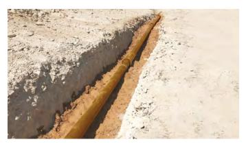
Flowstrong GRE Pipes & Fittings Diameter Range (DN): 3" - 16" Pressure Class (PN): Up to 3000 psi Standard Lengths: 6 - 12 m
